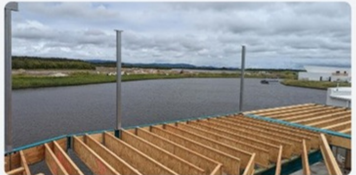
Deck & Structure Framing
