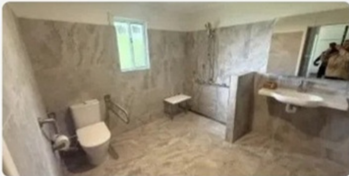
Bathroom Renovation & Reinstatement
